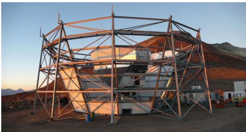
The Atacama Cosmology Telescope under construction in the Chilean Andes
